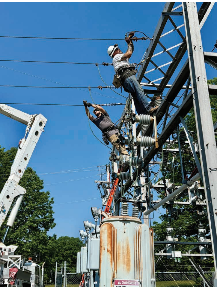
SUBSTATION WORK: United Electric Apprentice Lineman Spencer Pomerleau, left, and Journeyman Lineman Keegan Prisk re-attach connections in the Graham substation during a planned outage. These outages ensure the safety of our employees and members during the line work.
