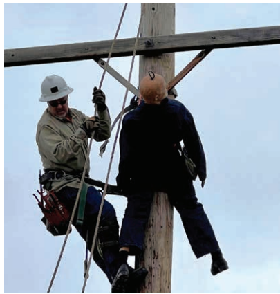
LIFE-SAVING TRAINING: Crew Chief Carl Yebernetsky prepares to lower a training dummy safely to the ground for his yearly pole-top rescue certification. Safely climbing a pole to reach an incapacitated fellow lineworker is a procedure all lineworkers must learn. This and other ongoing training help to instill trust among coworkers in emergency situations.
